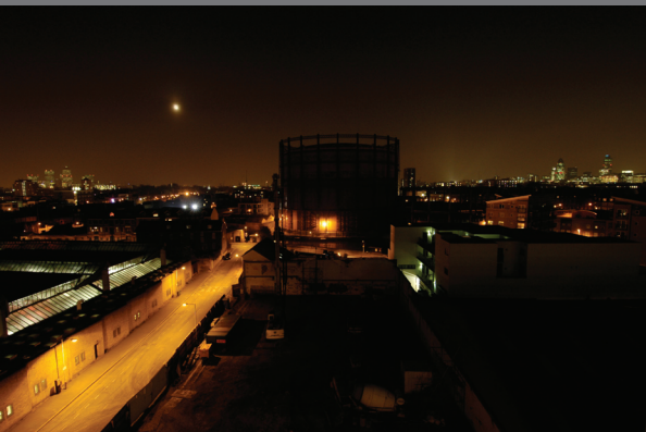
Imperial Gas Works, 21 March
